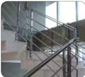
Grade 430 welded tube
