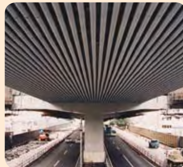
Overpass noise-absorbing plate, Japan.
