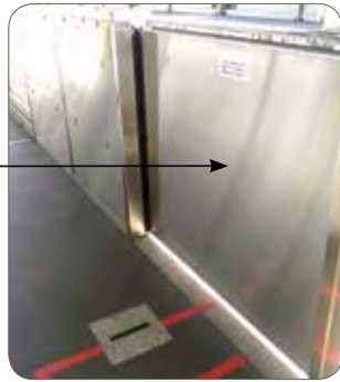
Railway station safety barrier, in SUS430JL, Japan.
