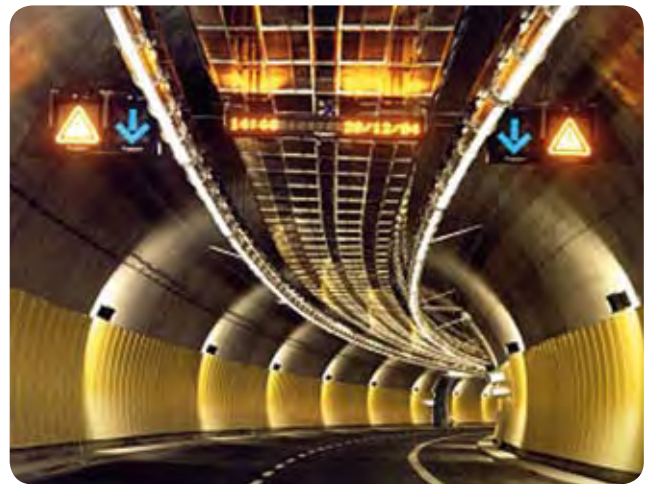
Cladding panels, in coated grade 430, Italy.
