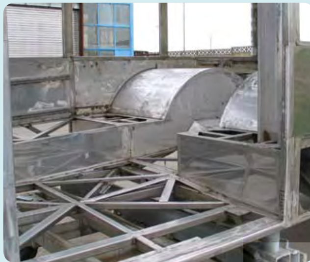
Welded structural frame in grade 1.4003.
